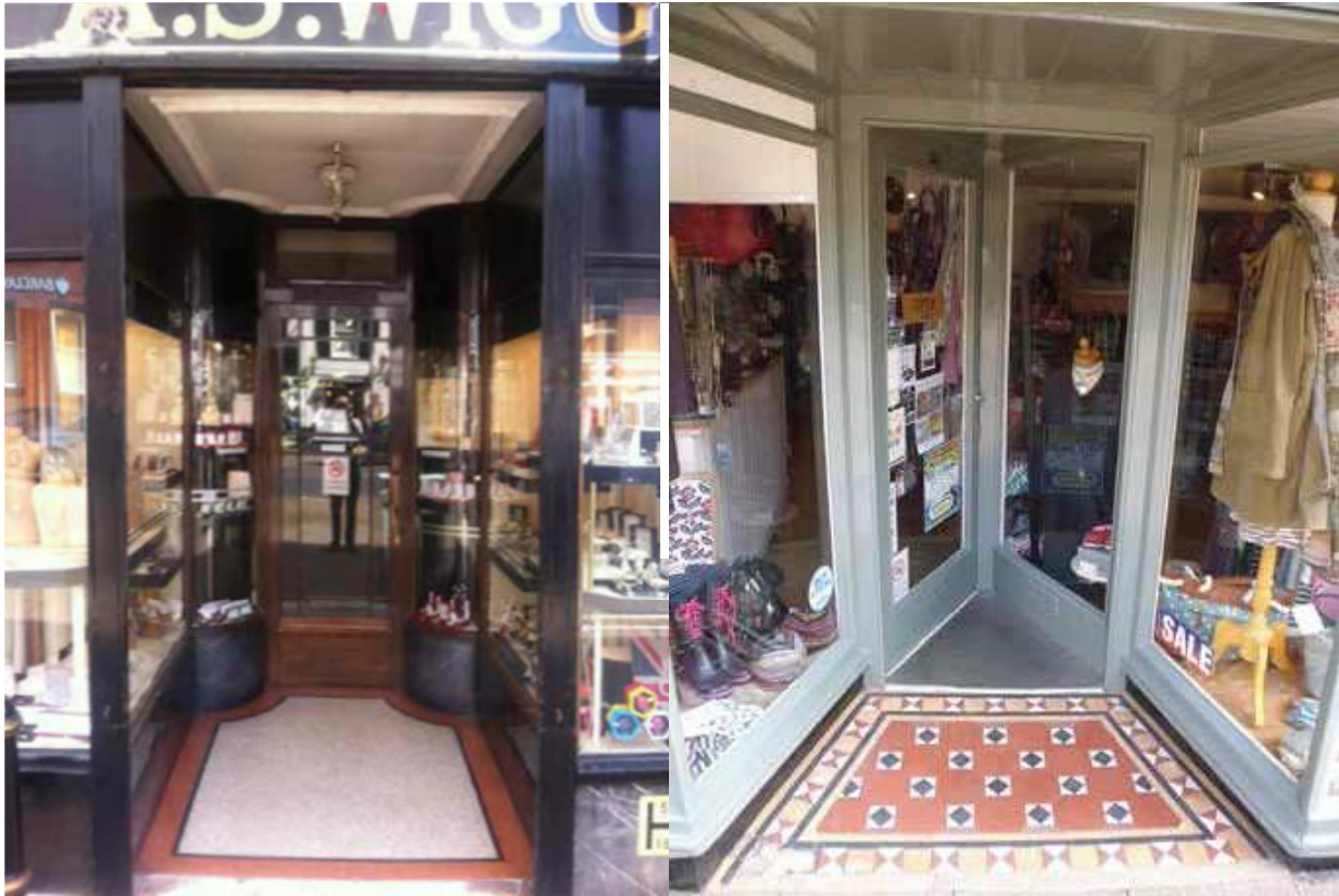
Well designed entrance: recessed, level access and outward opening
