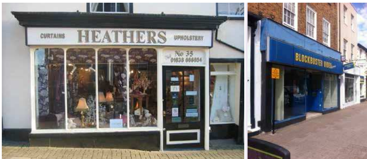
Traditional designed shop front retaining original detail
