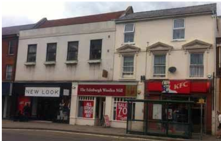
Shopfront straddling two buildings
