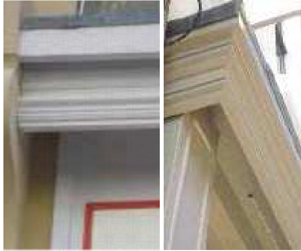
Cornice incorporating recessed lighting
