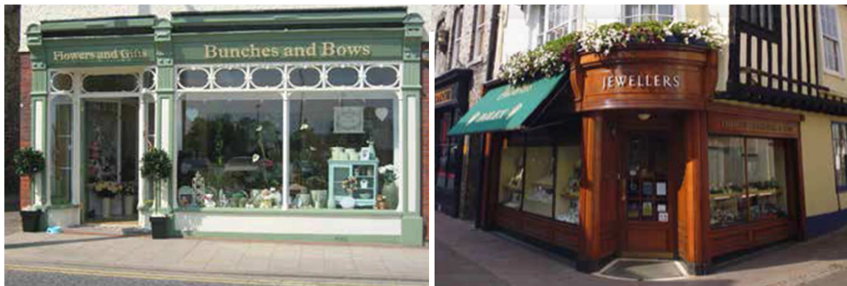
Examples of traditionally designed shopfronts retaining original detail
